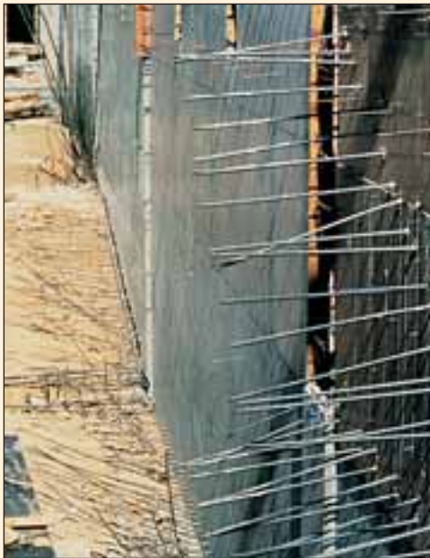
Exposed dowels on the job site are a hazard. In addition, they can be bent or damaged.
