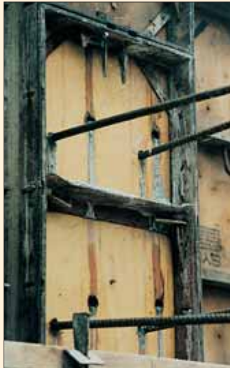
Drilling forms for dowels is expensive, and form removal is difficult and time consuming.
