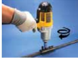
2) Tighten bolts from the center to the end to secure onto the first reinforcing bar.
